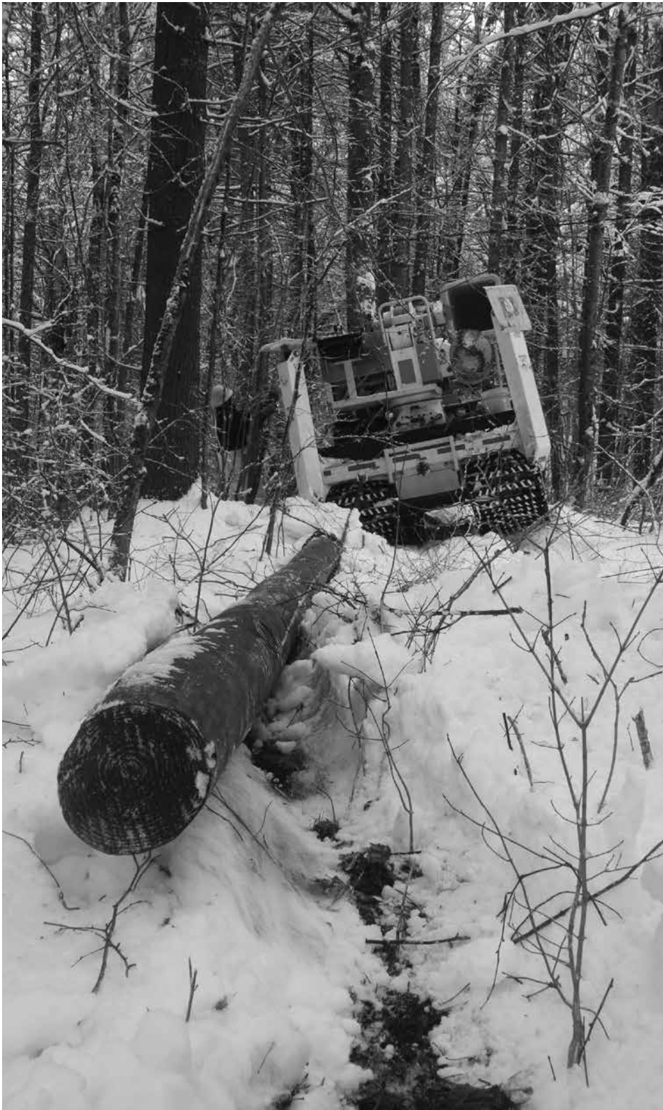
There are lots of places on WEC’s system that you can’t reach by truck. In these photos Hans Pope-Howe, with Donnie Singleton guiding him, drags a new pole into the woods behind WEC’s track vehicle to replace a pole (middle below) whose top had snapped off and was dangling from the conductor.
