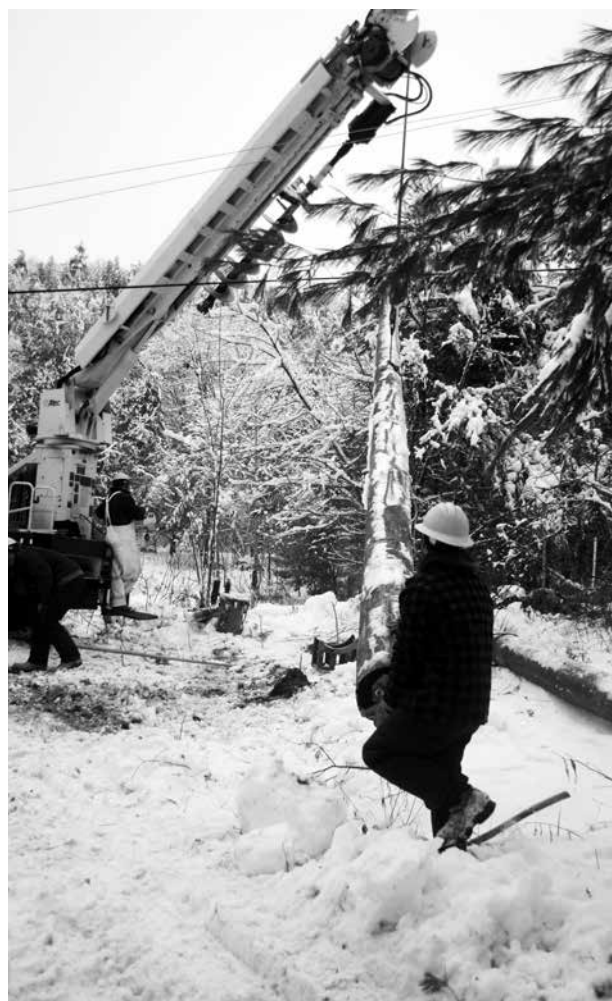
In this set of photos, the team of Doug deGroseilliers (checked coat), Donnie Singleton, and Hans Pope-Howe replace a broken pole by a member’s driveway in Tunbridge. With Donnie operating the derrick controls on the back of the truck, which hoists the new pole off the ground, Doug guides the base toward the hole that’s been prepared for it. In center photo, Hans is perched in a bucket (attached to WEC’s track vehicle), stabilizing the top of the pole.
