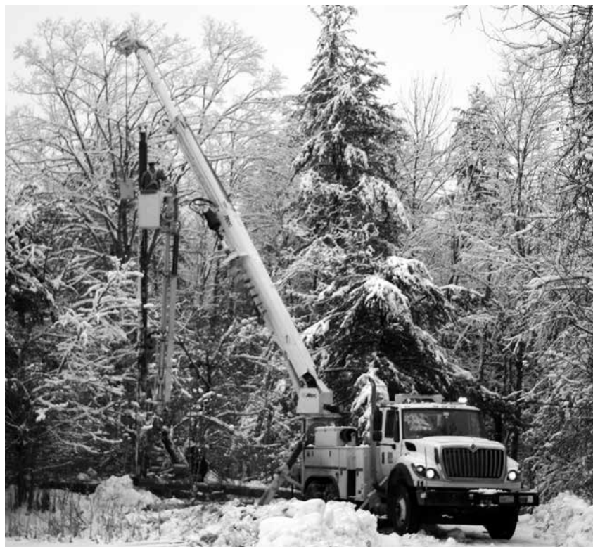
In this set of photos, the team of Doug deGroseilliers (checked coat), Donnie Singleton, and Hans Pope-Howe replace a broken pole by a member’s driveway in Tunbridge. With Donnie operating the derrick controls on the back of the truck, which hoists the new pole off the ground, Doug guides the base toward the hole that’s been prepared for it. In center photo, Hans is perched in a bucket (attached to WEC’s track vehicle), stabilizing the top of the pole.
