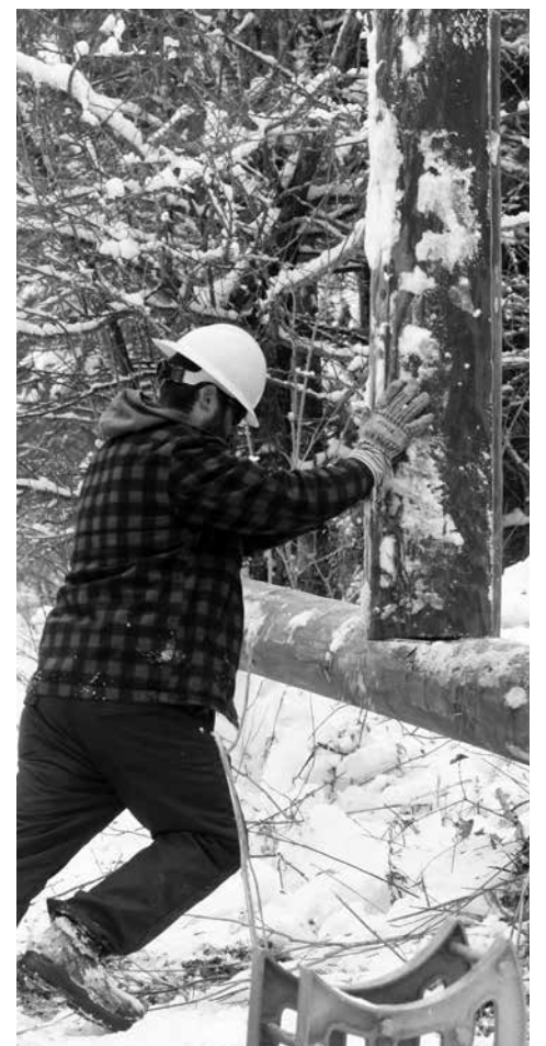
In this set of photos, the team of Doug deGroseilliers (checked coat), Donnie Singleton, and Hans Pope-Howe replace a broken pole by a member’s driveway in Tunbridge. With Donnie operating the derrick controls on the back of the truck, which hoists the new pole off the ground, Doug guides the base toward the hole that’s been prepared for it. In center photo, Hans is perched in a bucket (attached to WEC’s track vehicle), stabilizing the top of the pole.
