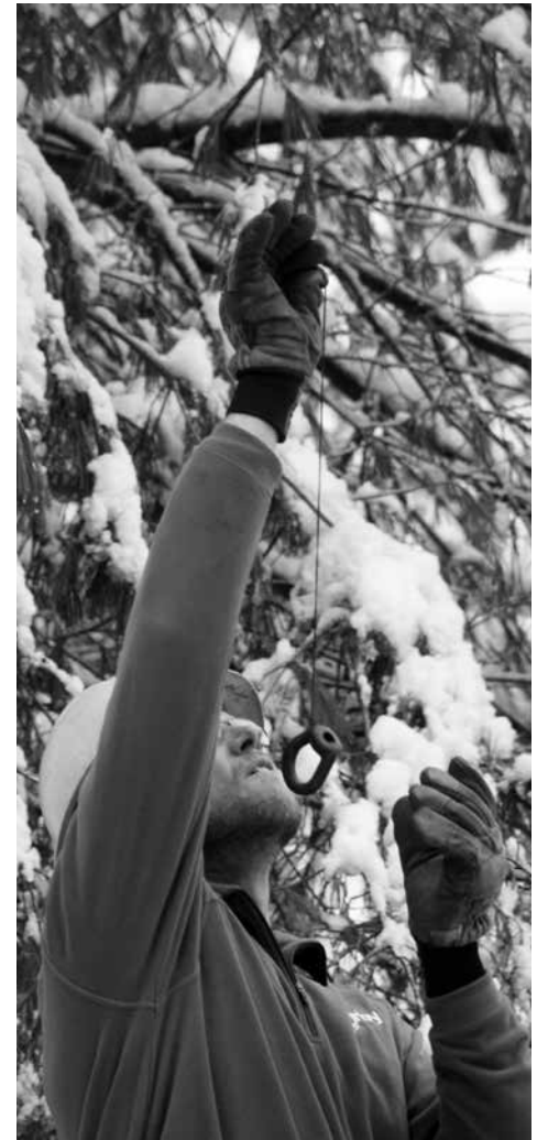
(Left) There’s a power line in there somewhere. In one of WEC’s hardest-hit areas, off of Larkin Road in Tunbridge, there were hardly any unscathed spans of line. At right, Hans Pope-Howe dangles a plum line to check whether a newly set power pole is straight and vertical.
