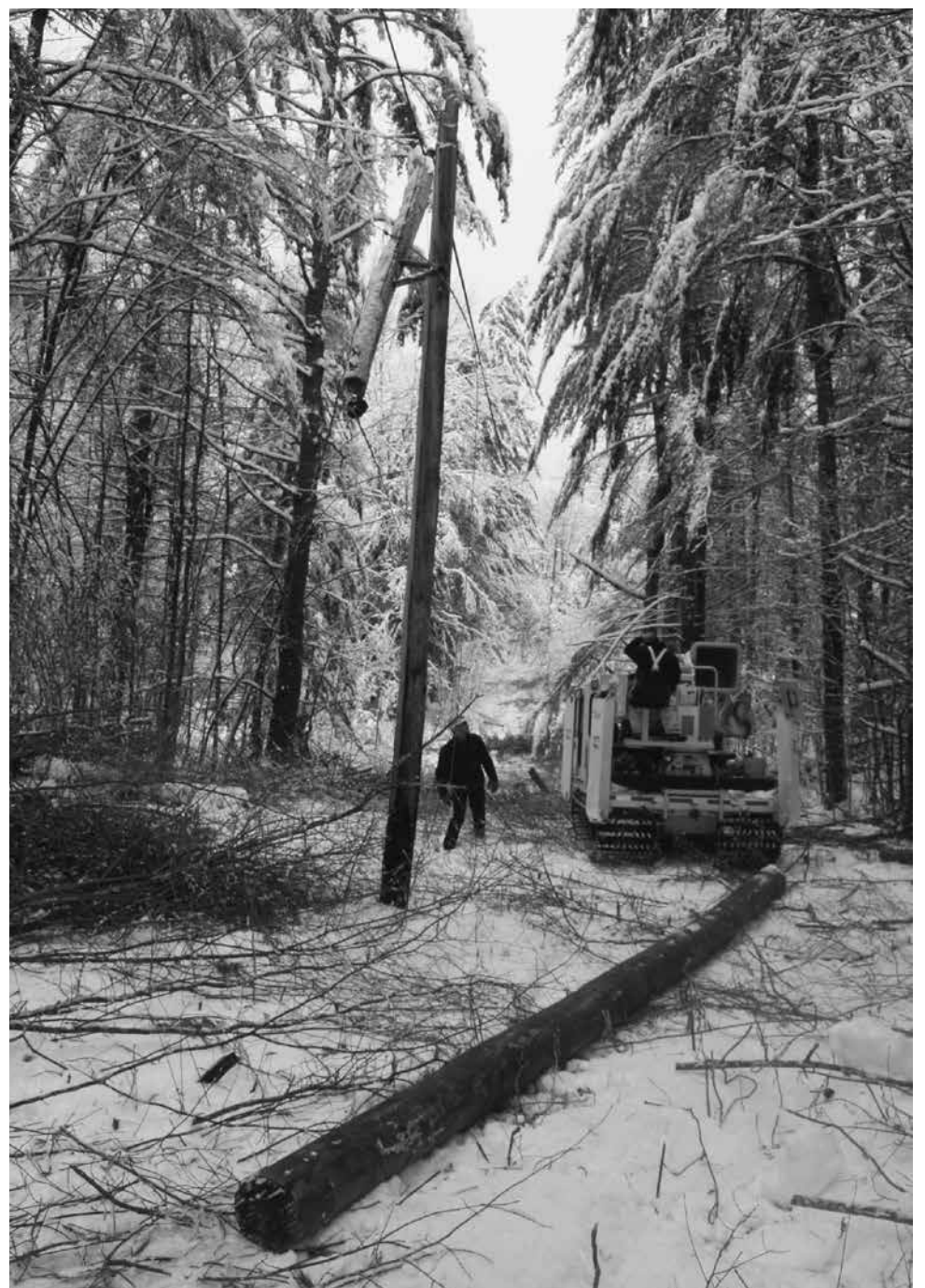
There are lots of places on WEC’s system that you can’t reach by truck. In these photos Hans Pope-Howe, with Donnie Singleton guiding him, drags a new pole into the woods behind WEC’s track vehicle to replace a pole (middle below) whose top had snapped off and was dangling from the conductor.
