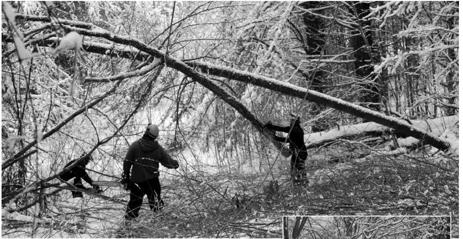
Above, a contracted right-of-way clearing crew sets about the task of cutting broken trees off the power lines in an off-road corridor in Tunbridge. As this photo shows, much of the storm's damage came from trees that fell in from outside the right-of-way. At right, First Class Line Worker Doug deGroseilliers (left) and Equipment Operator Donnie Singleton connect the primary conductor of a sagging line to the neutral, making it safe for the tree crew to do its work.
