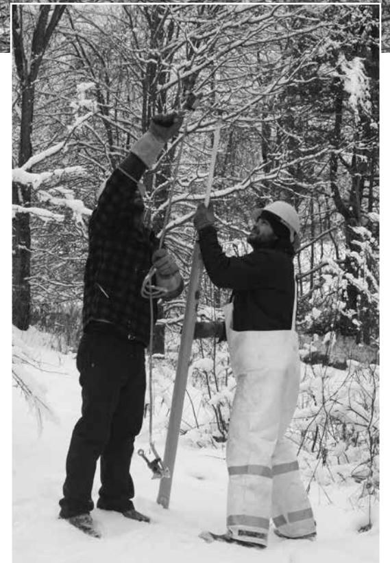
Above, a contracted right-of-way clearing crew sets about the task of cutting broken trees off the power lines in an off-road corridor in Tunbridge. As this photo shows, much of the storm's damage came from trees that fell in from outside the right-of-way. At right, First Class Line Worker Doug deGroseilliers (left) and Equipment Operator Donnie Singleton connect the primary conductor of a sagging line to the neutral, making it safe for the tree crew to do its work.
