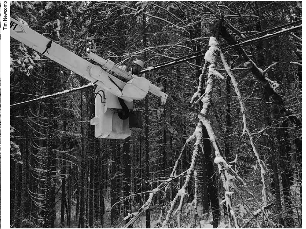
The power – and danger – of heavy snow. In Worcester, Tim Newcomb captured a snowy tree limb dangling over a power line – in the very area Right of Way crews trimmed after the October 2017 windstorm. Sometimes heavy snow bends a tree outside the ROW so far over it becomes an unexpected hazard to the lines. At right, crews at work repairing an outage caused by a broken limb on Minister Brook Road in Worcester.
