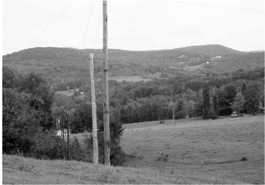
Sometimes the best option is to reconstruct rural and remote rights-of-way where they already are. It wasn't easy to reach these lines in Tunbridge, but the upgrade is easy to see: larger poles and a more resilient system than what had been in place. The old poles shown here still supported telephone lines, waiting to be moved by the telephone company to the new utility poles.
