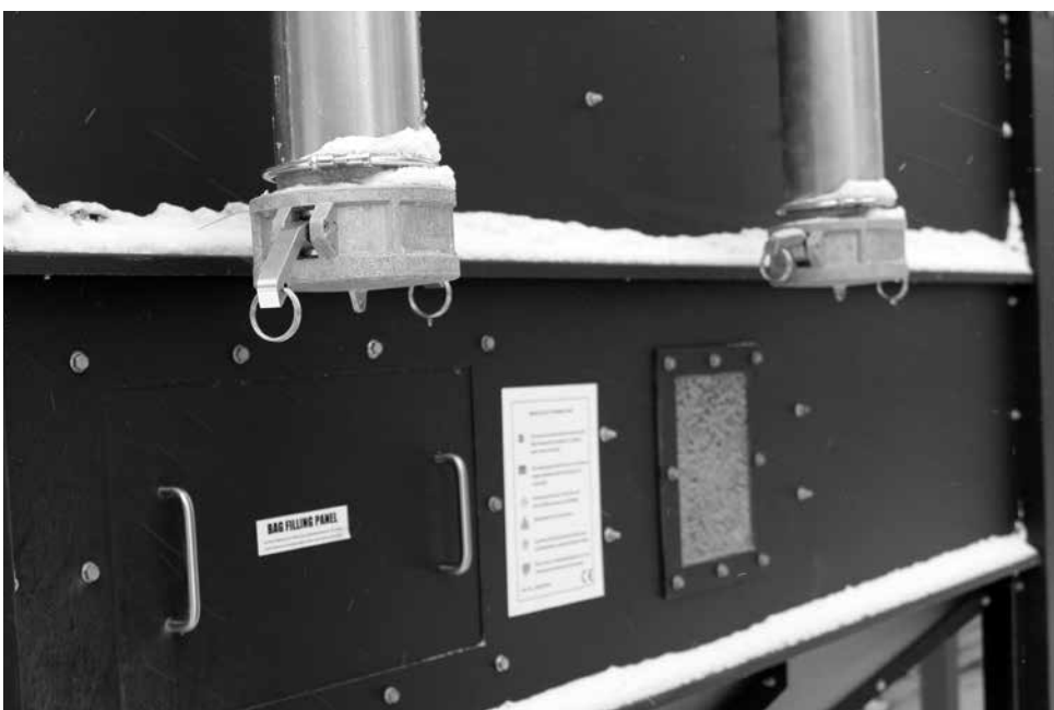
The outdoor bin’s pipes connect to the delivery truck; pellets are vacuum forced into the bin. A window shows the pellet level.
