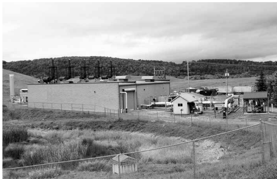
WEC's power plant at Coventry Landfill harvests landfill gas to create stable, inexpensive electricity that powers two thirds of WEC members' homes. While the phrase "renewable" seems strange applied to garbage gas, WEC puts a landfill byproduct to good use.
