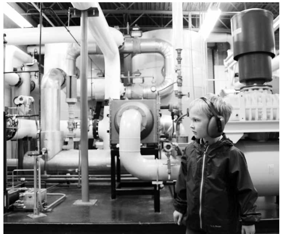
Coventry had its highest performing year ever, supplying enough power to keep the lights on in 75 percent of WEC households. Here, a young visitor tours the landfill gas-to-energy plant in 2019.
