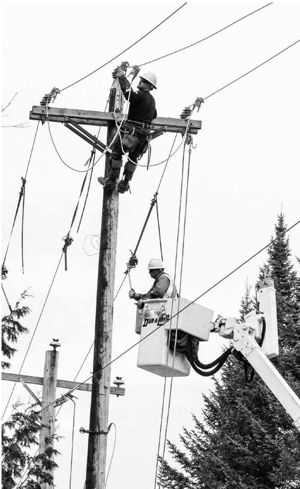
WEC lineworkers lift power lines to accommodate broadband rollout.
